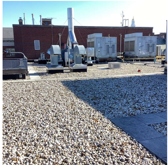
Roof 1 - East View
