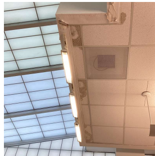
Skylight - Room 100A
