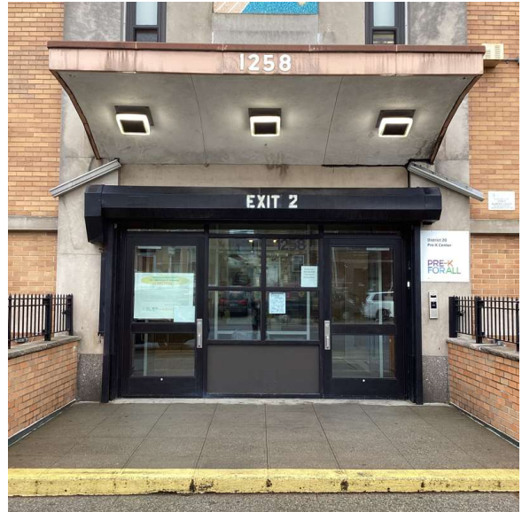
Facade A - 65th Street
