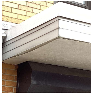
Facade A No violations recorded.
