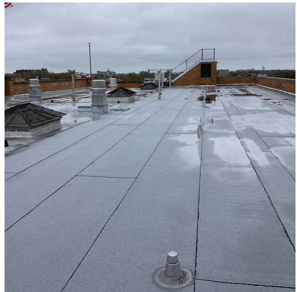
Roof 1 - Southeast View
