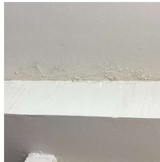
Roof 1 - Stairwell B/3 (Roof 2 - Multipurpose Room Stage similar)
