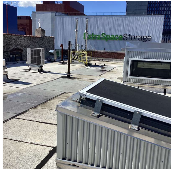
Roof 1 - Northeast View
