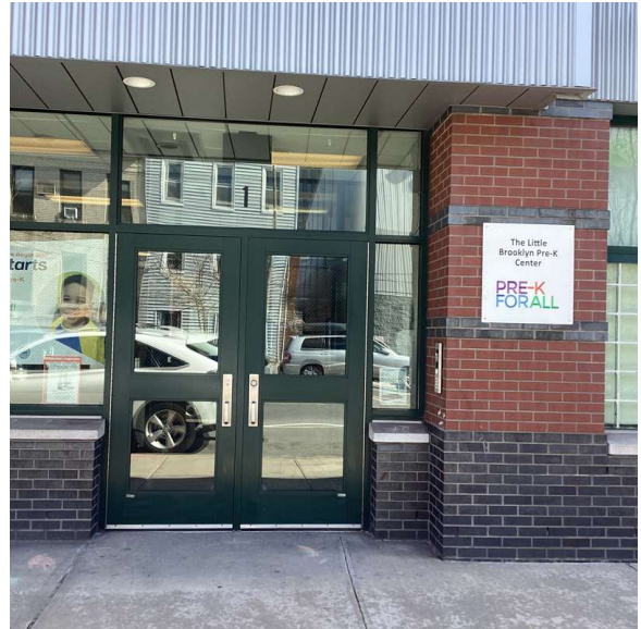
Facade A - 3rd Avenue
