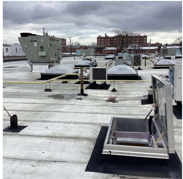
Roof 1 - East View
