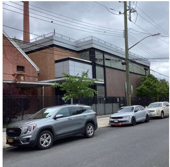
West 35th Street - Southeast View
