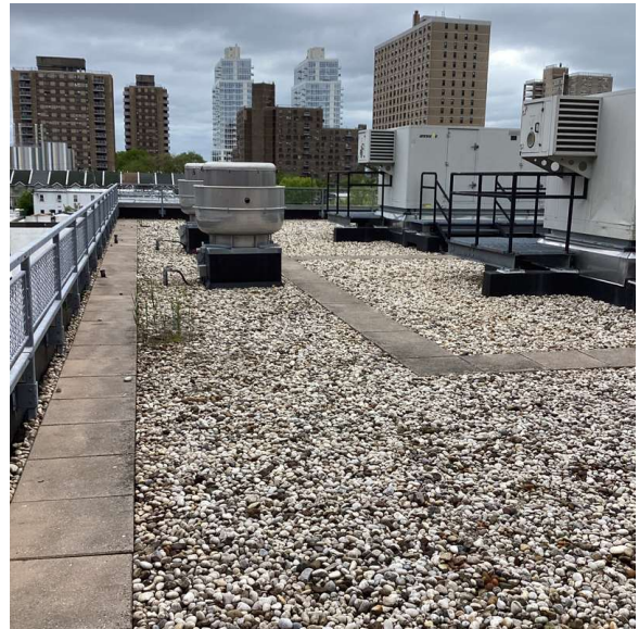
Roof 1 - South View
