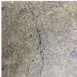
Facade A No violations recorded.
