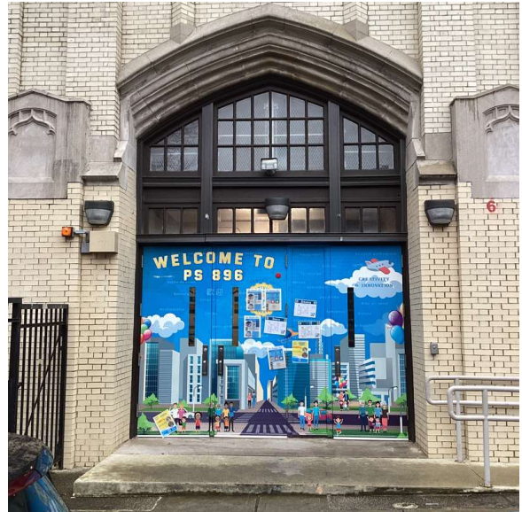
Facade A - Southwest View
