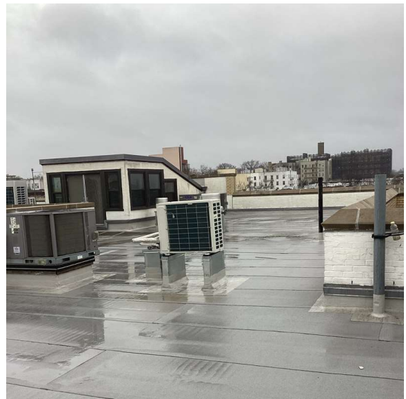
Roof 1 - North View
