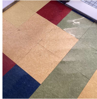
Corridor near Students Toilets Rooms - 3rd Floor
