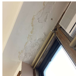
Facade H - Room 15
