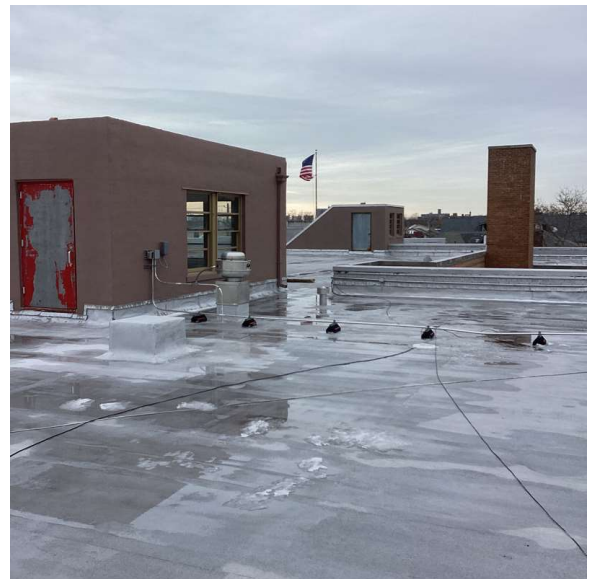
Roof 1 - Southwest View
