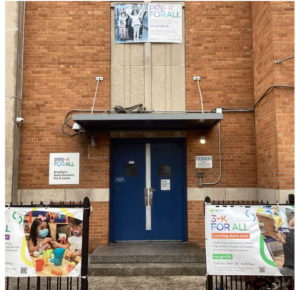
Facade A - Avenue W
