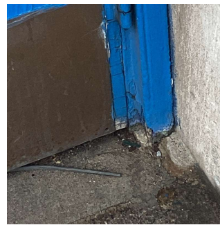
Facade H No violations recorded.
