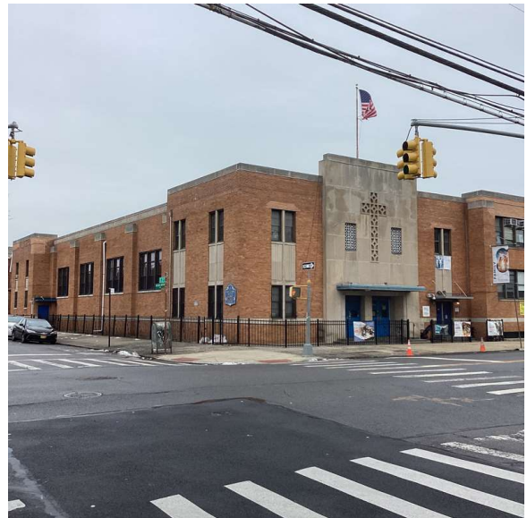
Corner of Avenue W and East 2nd Street - Northeast View
