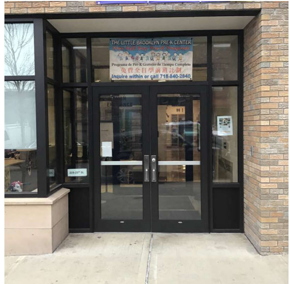
Facade A - 25th Street
