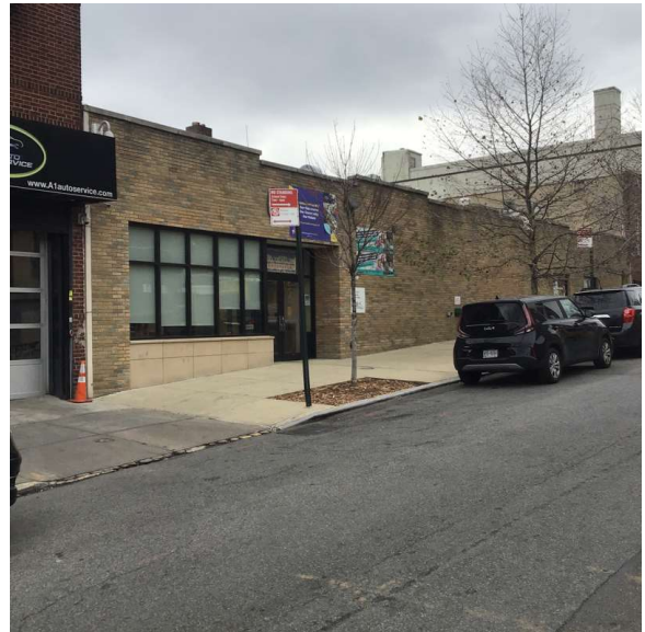
25th Street - East View
