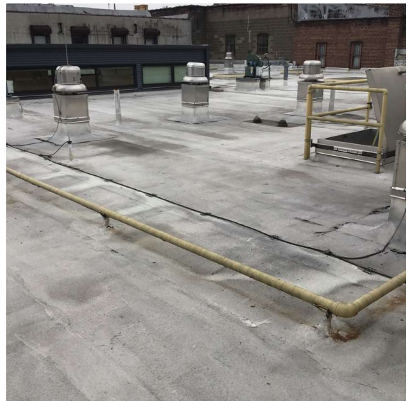
Roof 1 - North View
