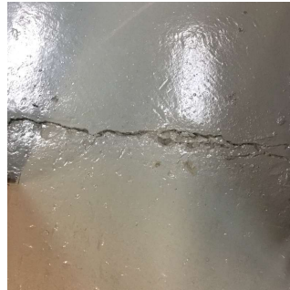
Room B64 (Room B43, Basement Corridor, Custodian Shop similar)
