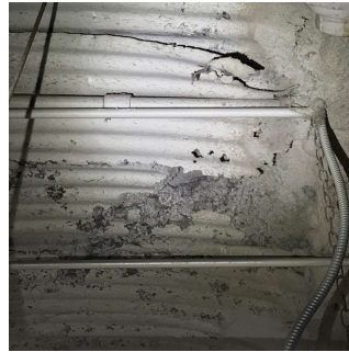
Basement Storage Area
