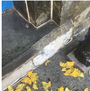
Facade D - Exit 4 No violations recorded.
