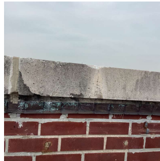
Roof 1 - Near the Bulkhead
