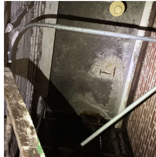
Basement - Vault next to the sidewalk elevator
