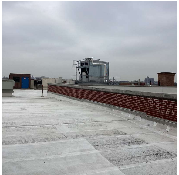
Roof 1 - Southwest View
