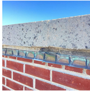
Roof 1 - Facade F
