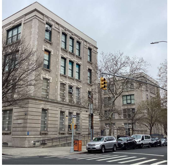
Corner of Albany Avenue and Bergen Street - Northwest View
