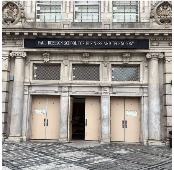
Facade A - Albany Avenue
