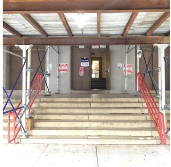
Facade A - Wells Street
