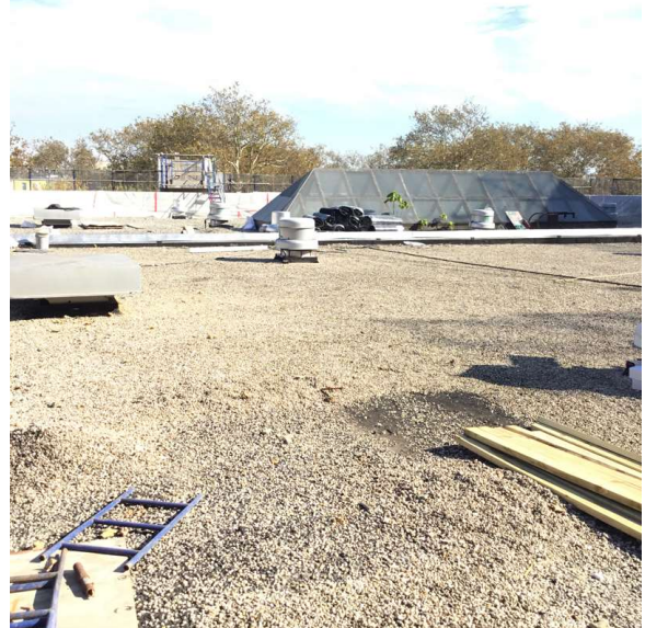
Roof 5 - Southeast View
