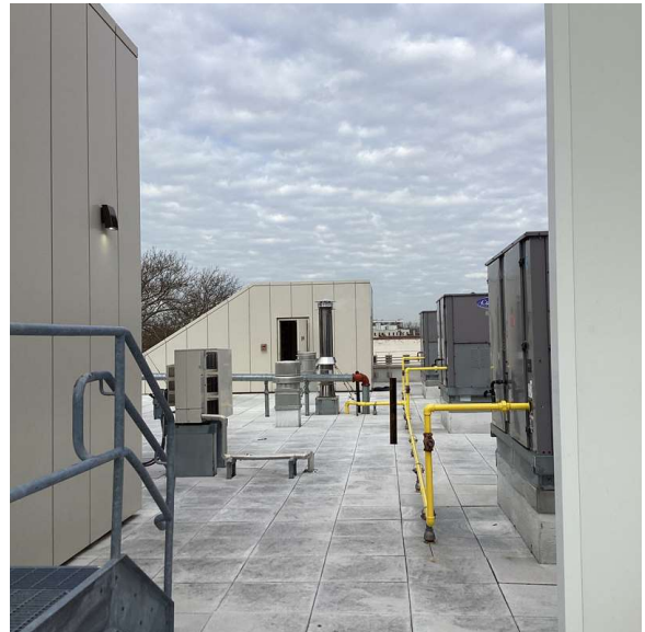
Roof 1 - Northwest View
