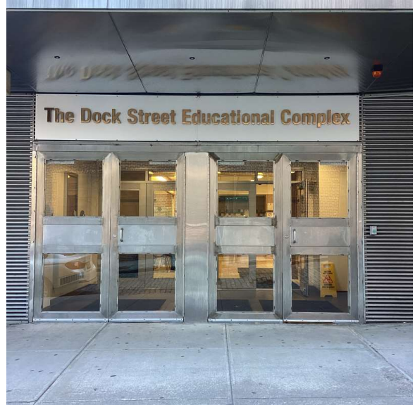
Facade A - Dock Street
