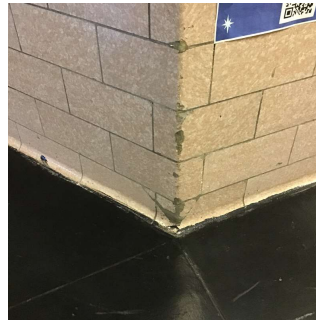
Corridor near Room 338
