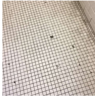
Boys Locker Room
