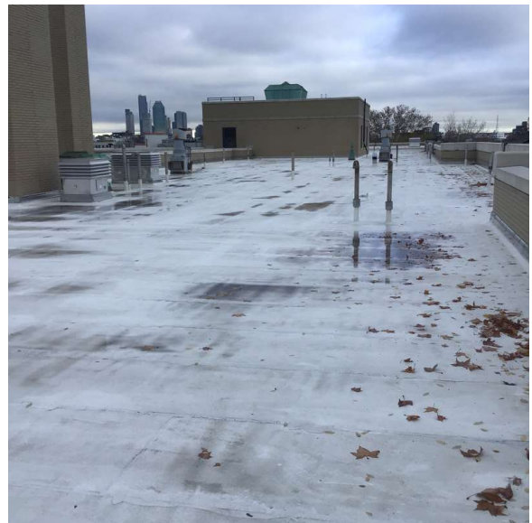
Roof 1 - North View
