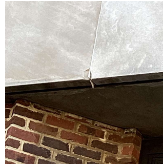
Facade A - Near AW1
