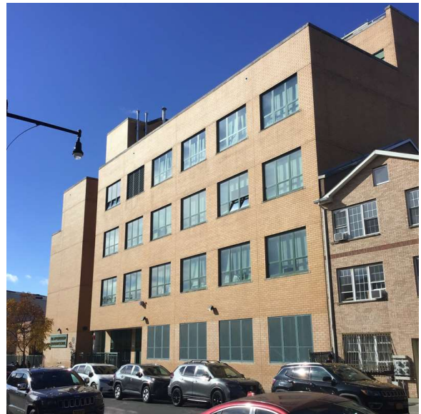
Palmetto Street - Southwest view
