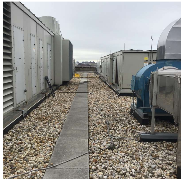
Roof 1 - Southwest view
