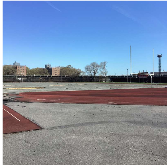
Football/Soccer Field - East view
