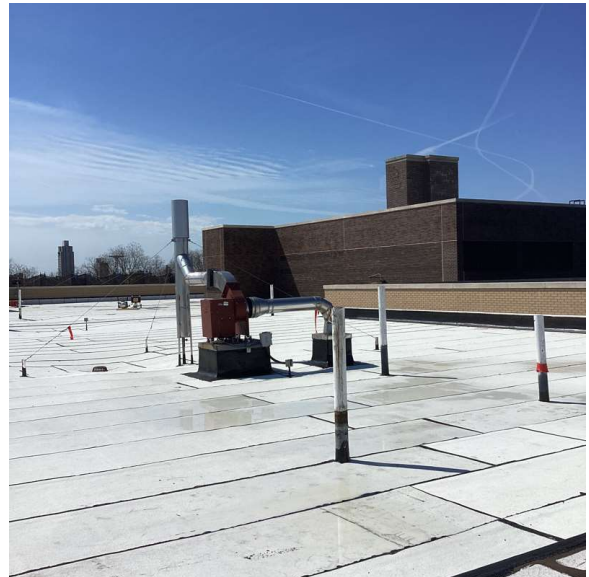
Roof 1 - Southwest view
