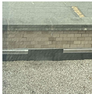
Roof 4 - Facade J
