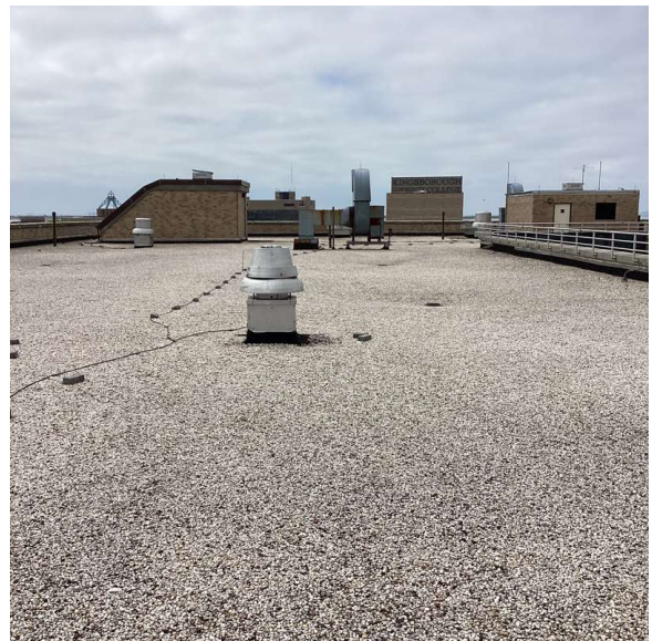
Roof 1 - South View
