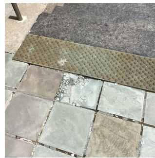
Facade D No violations recorded.
