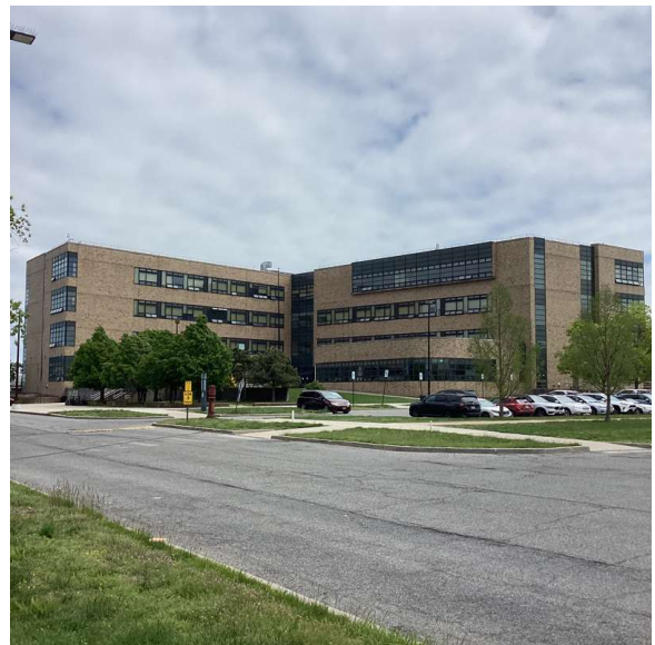
Shore Boulevard - Southeast View
