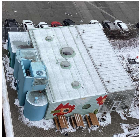
All Roofs - Southeast View
