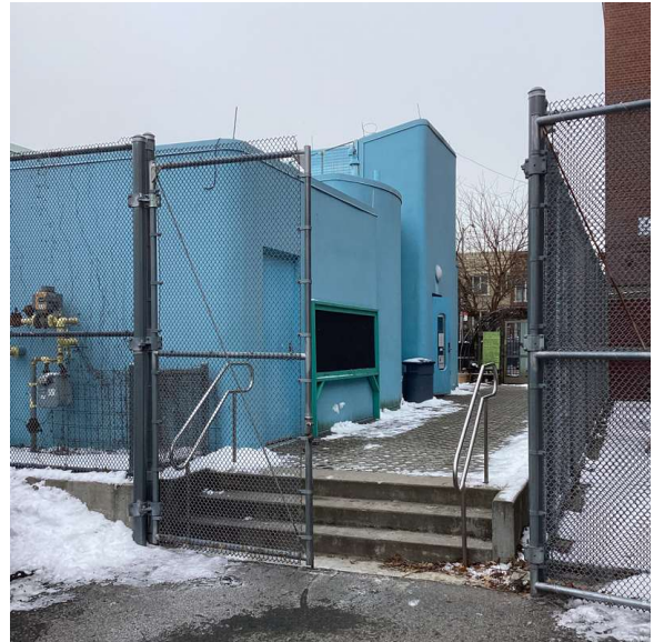
Facade A - Southwest View
