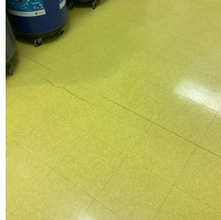
Corridor near Room C07 No violations recorded.
