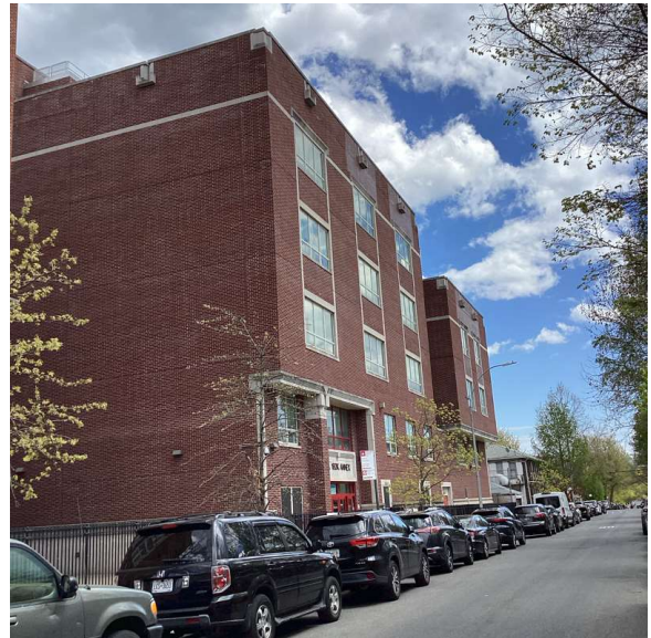
52nd Street - East View
