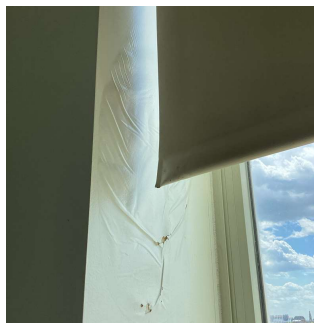
Facade A - Rooms 415 (Shown), 505, 509, Facade F - Room 122, 316, 414, 416, Library similar
