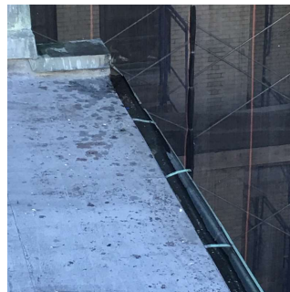
Gutter - Facade D No violations recorded.
