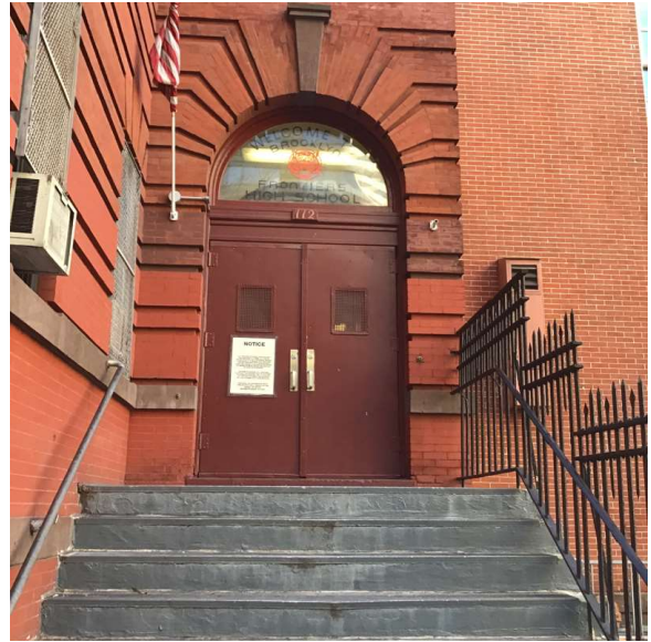
Facade A - Schermerhorn Street
