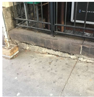
Facade A No violations recorded.
