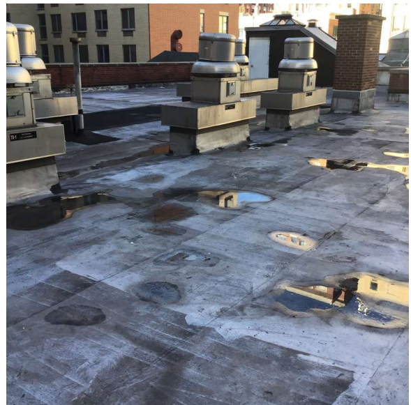
Roof 1 - West View
