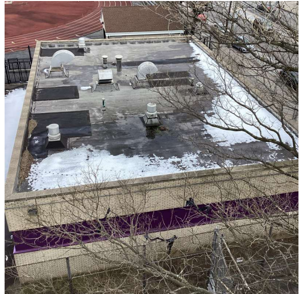
Roof 1 - Northeast View
