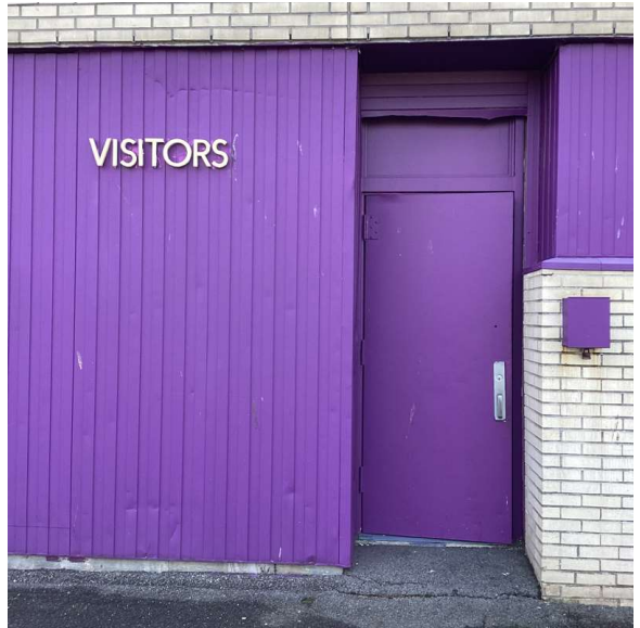
Facade C - Field House
