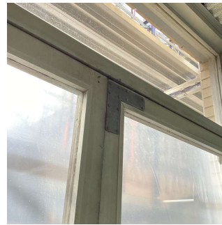
Exit to Courtyard near Room 157 No violations recorded.
