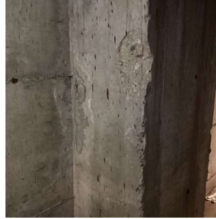
Crawlspace near the Stair F No violations recorded.
