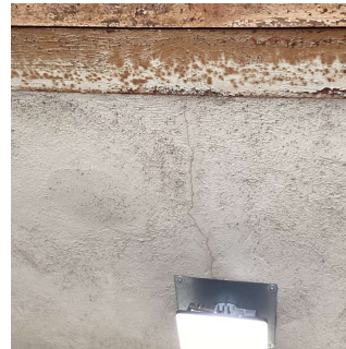
Facade K - Exit 9A
