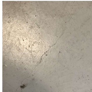
3rd Floor - Room 340 No violations recorded.
