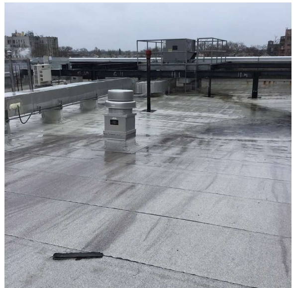
Roof 1 - Northeast view
