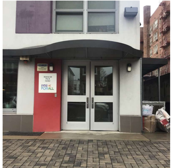
Facade A - 71st Street
