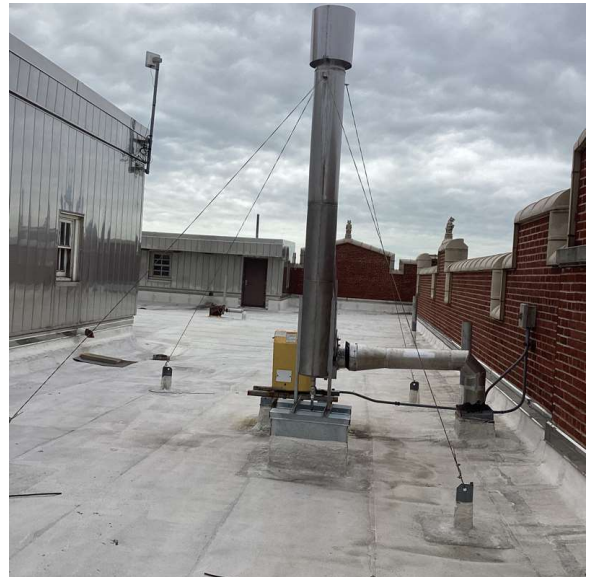
Roof 1 - Southeast View
