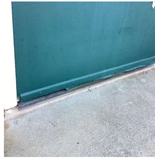
Facade A - Main Entrance
