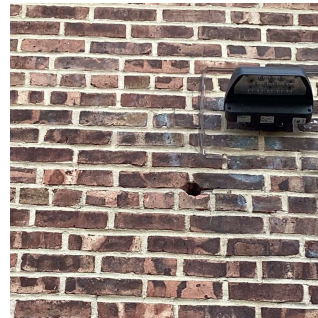
Facade B - Near Exit 2/3
