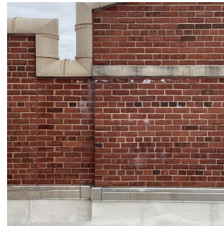
Roof 1 - Facade C No violations recorded.
