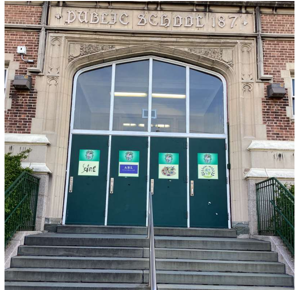
Facade A - 65th Street
