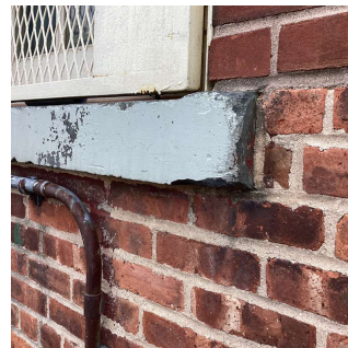
Facade G - Near Exit 9
