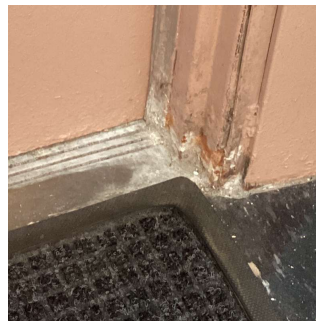
Facade B - Exit 2/3
