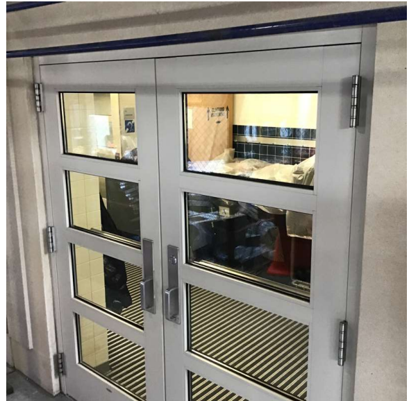
Facade A - 30th Street
