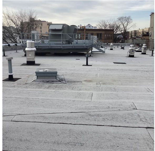
Roof 1 - South View
