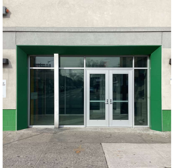
Facade A - Flatbush Avenue
