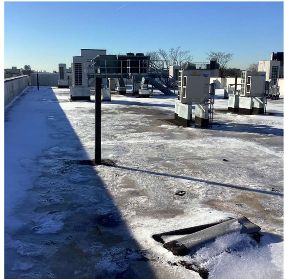
Roof 1 - Southwest View
