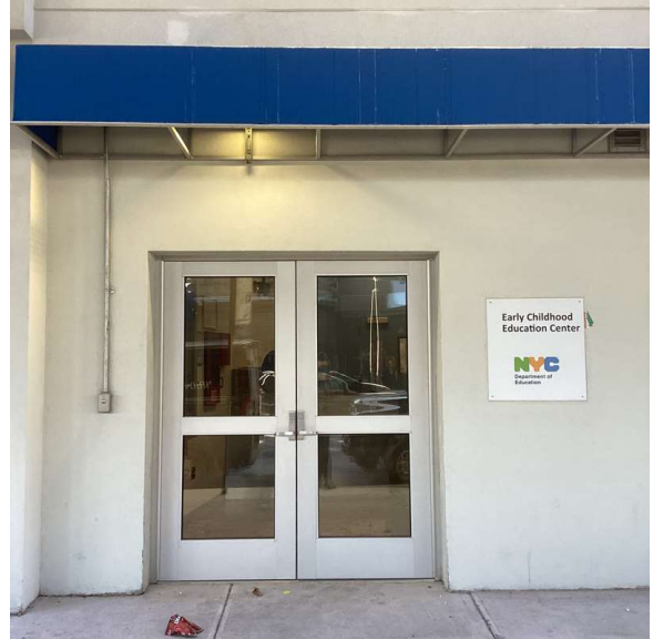
Facade A - New Utrecht Avenue
