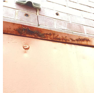
Plaza Deck - BH3
