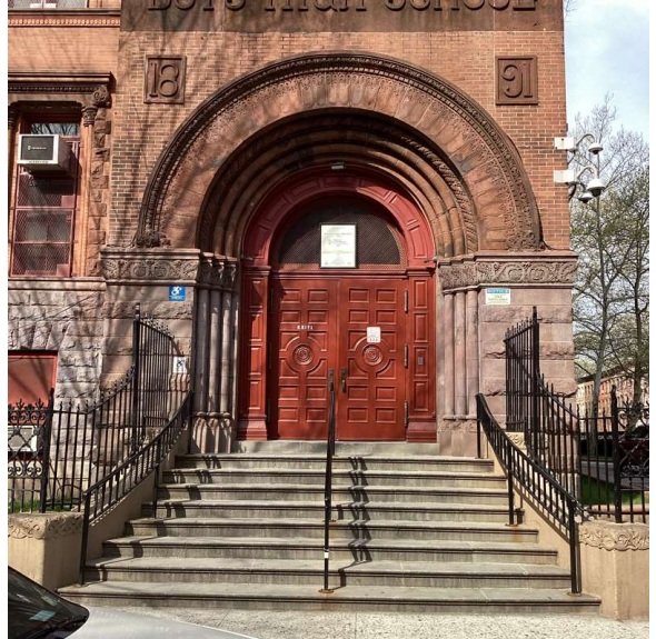
Facade A - Marcy Avenue
