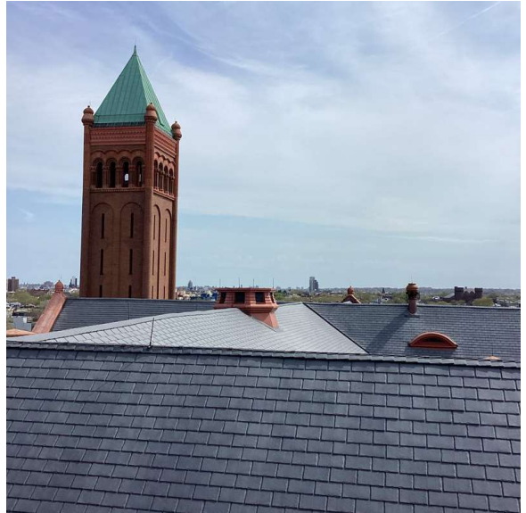
Roofs 1, 2, 3 - Northeast View
