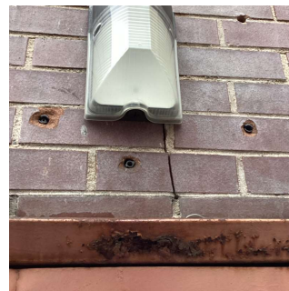
Plaza Deck - BH3
