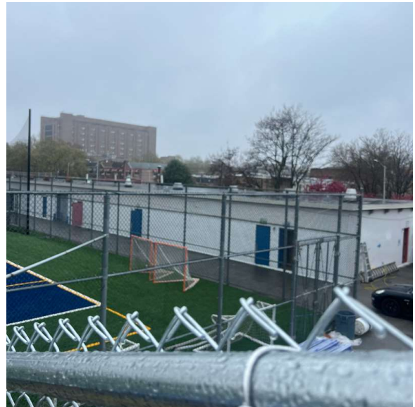
Roof 1 - Southeast View
