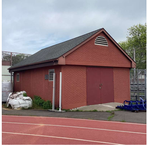
Corner of Facade A and B - Northwest View
