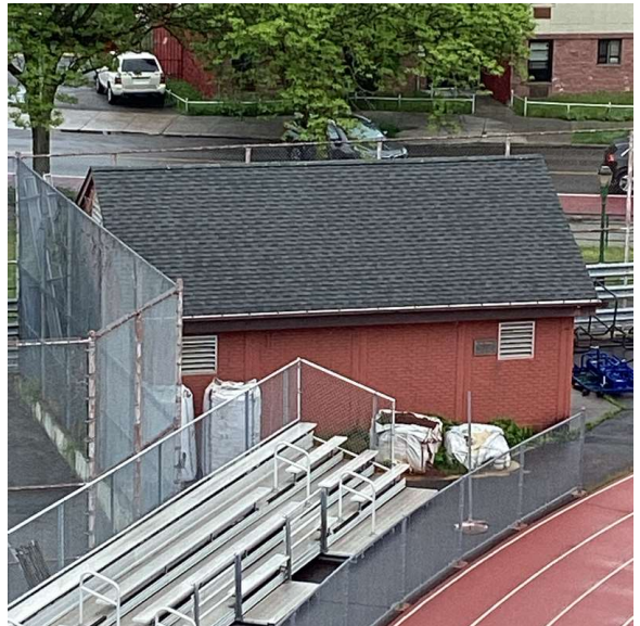
Roof 1 - Southeast View
