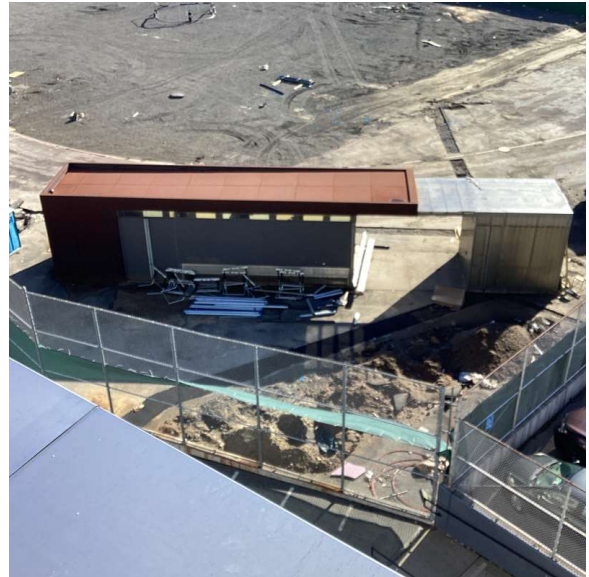
Roof 1 - Southeast View
