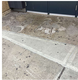
Exit 7 - Facade R
