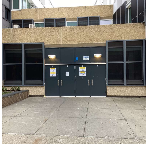
Facade A - Grand Street
