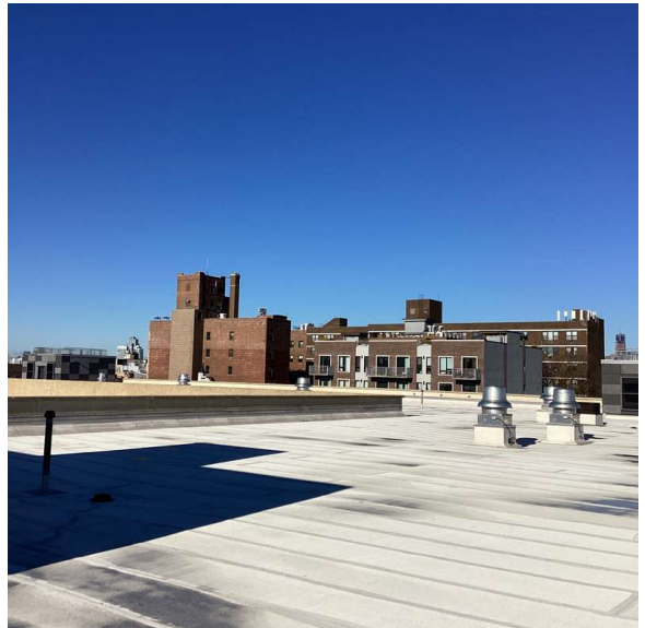
Roof 1 - West View
