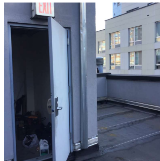
Penthouse No violations recorded.
