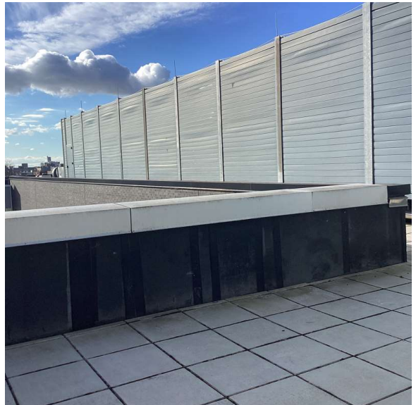
Roof 1 - South View
