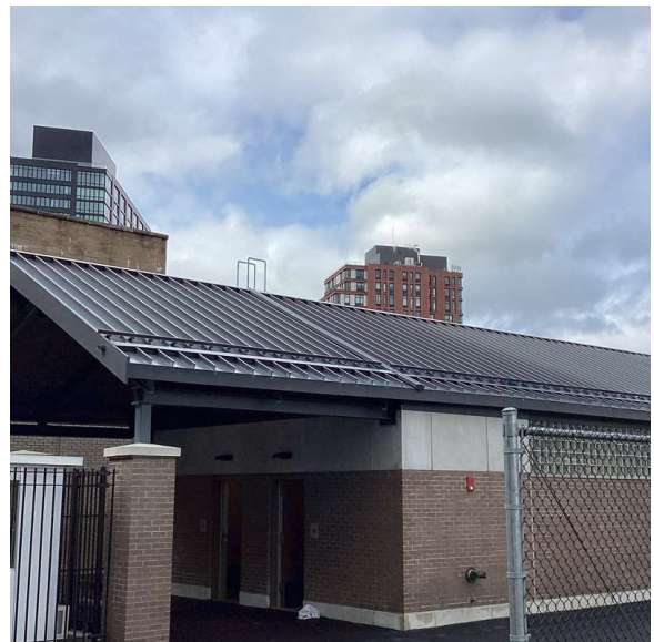
Roof 1 - Southwest View
