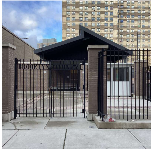
Facade A - Clermont Avenue
