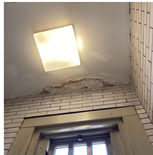
Roof 1 - 1st Floor - in West Office Room No violations recorded.
