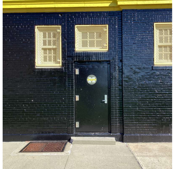
Facade A - Fieldhouse
