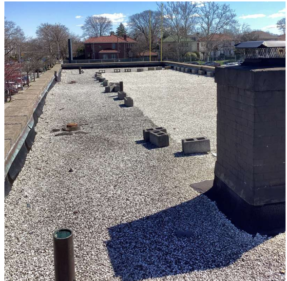
Roof 1 - Northeast View
