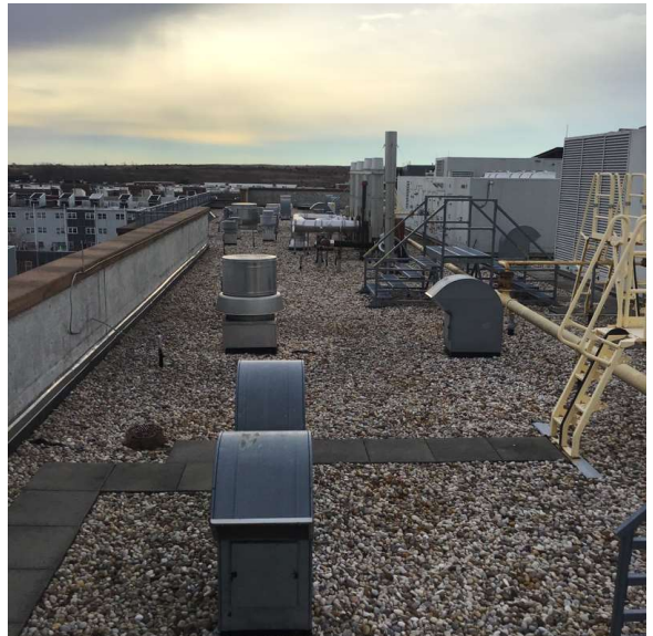
Roof 1 - Southeast view
