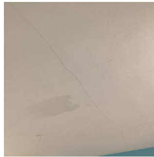
Corridor near Room 318A
