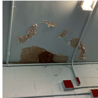
Roof 2 - Electrical Panel Room
