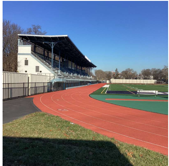
Grandstand/Fieldhouse - Northwest View
