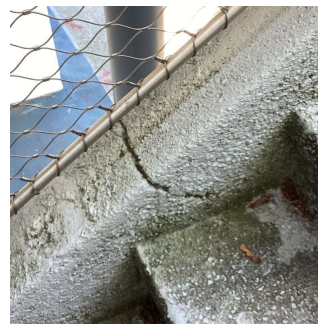
Facade D - Grandstand No violations recorded.
