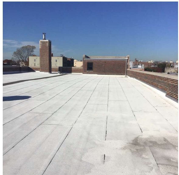
Roof 1 - West View
