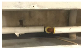
Electrical Room B110
