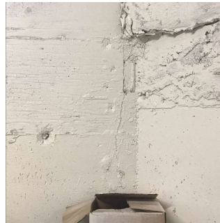
Electrical Room B110
