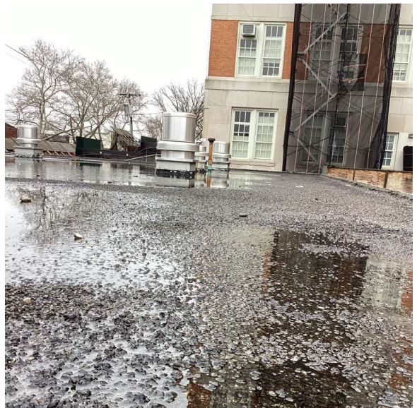
Roof 1 - North View
