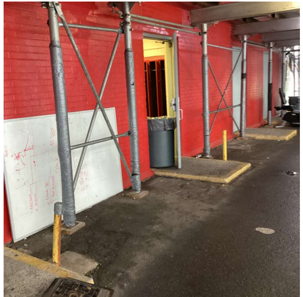
Facade A - Fieldhouse
