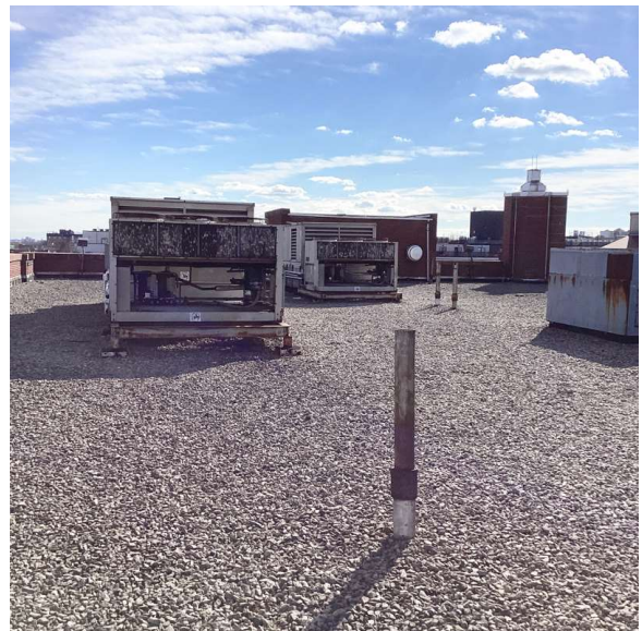
Roof 1 - East View
