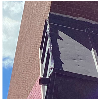
Roof 2 No violations recorded.
