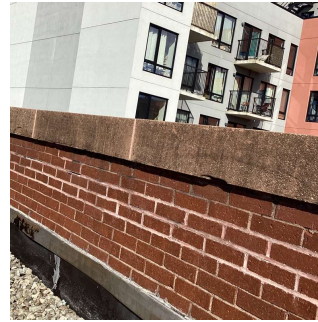
Roof 1 - Facade C
