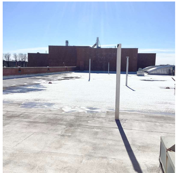
Roof 1 - South View
