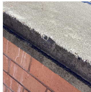
Roof 4 - Facade E No violations recorded.
