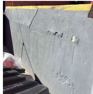
Facade F - Near Exit 15 No violations recorded.
