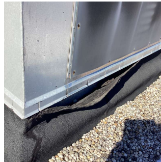
Roof 2 - Near Roof Hatch
