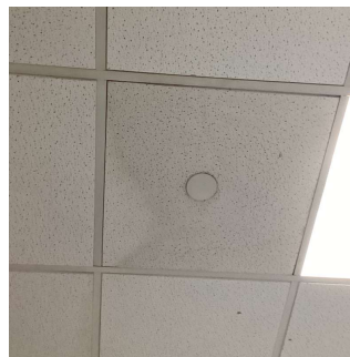
Roof 1 - Corridor near Room 309 (shown), Roof 4 - Room 324 (similar)
