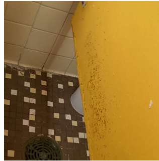
Inside Kitchen Women Locker Room
