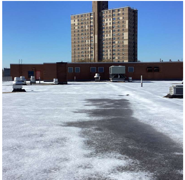
Roof 1 - West View
