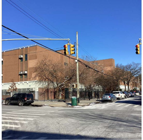
Corner of Troy Avenue and Maple Street - Northeast View
