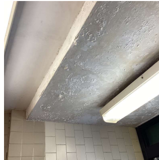
Stair B/Basement Vestibule
