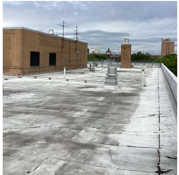
Roof 1 - Northwest View
